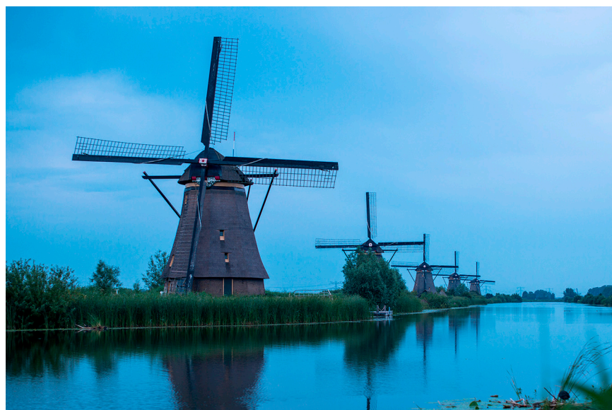
Low lands: Population pressure and generous investments made the Netherlands a pioneer in draining wetlands to create new land for agriculture. The iconic windmills now admired by tourists often served as pumps to remove water from low-lying areas. (Photo: R Boed/Flickr (CC BY 2.0 DEED).)
